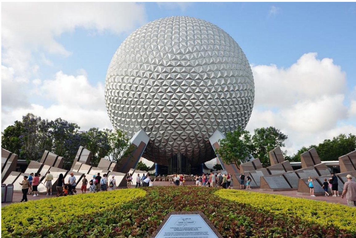
Figure 40: Spaceship Earth structure at Epcot Theme Park
